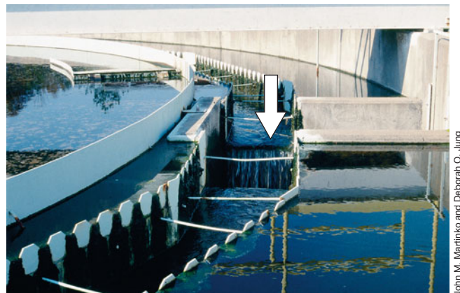
Figure 35.6 Primary treatment of wastewater. Wastewater is pumped into the reservoir (left) where solids settle. As the water level rises, the water spills through the grates to successively lower levels. Water at the lowest level, now virtually free of solids, enters the spillway (arrow) and is pumped to a secondary treatment facility.
